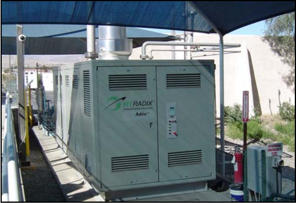
Figure 4. SunLine's HyRadix Adeo commercial reformer
