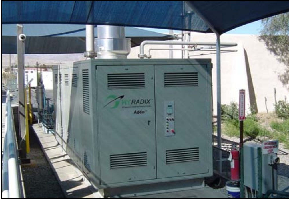
Figure 4. SunLine's HyRadix Adéo commercial reformer
