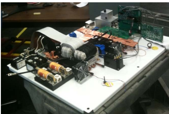
Figure 12. WPT system with AFE and isolation transformer. Copper foil wrapped inductor is part of the AFE and transformer in foreground with Litz windings.
