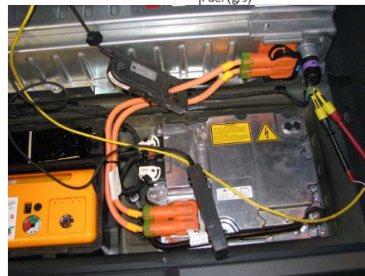
Figure 2. High-Voltage Battery and DC-DC Electrical Instrumentation.
