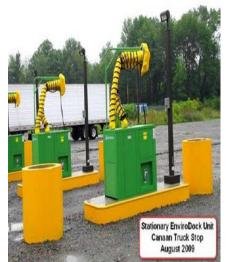
duplex power outlet for in-cab appliances, such as microwaves, computers, and coffee makers. Additionally, the E-Dock system also provides a duplex power plug on the outside unit itself for engine block heaters and any other power requirements.
