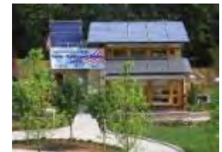
Renewable Energy Storage
