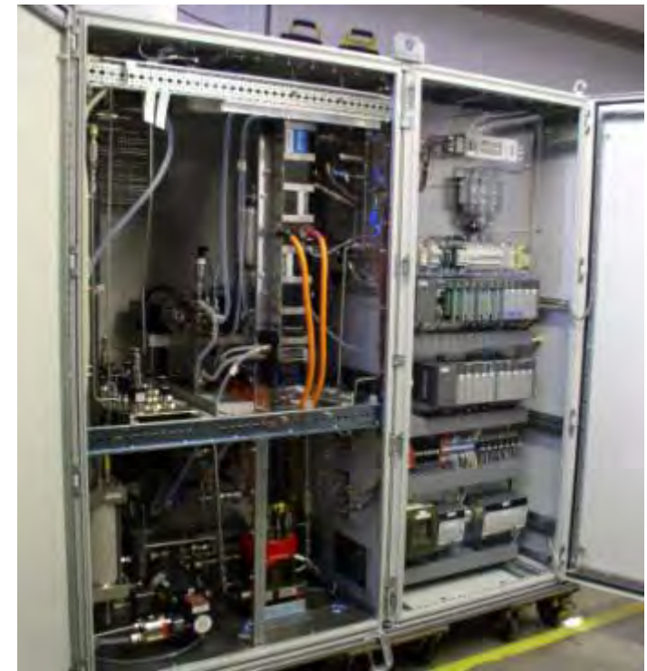
Proton's closed loop RFC system on test, demonstrating feasibility of UUV power concept
