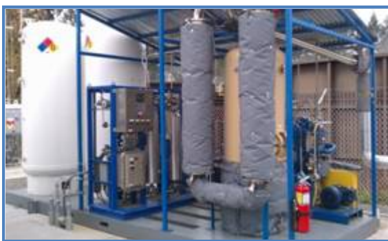
Wastewater biogas cleanup system at the Joint Base Lewis McChord (JBLM), near Tacoma, WA.
