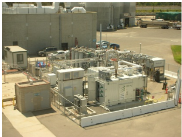
World's first trigeneration plant at the Orange County Sanitation District's WWTP in Fountain Valley, CA Photo from National Fuel Cell Research Center, UC-Irvine
