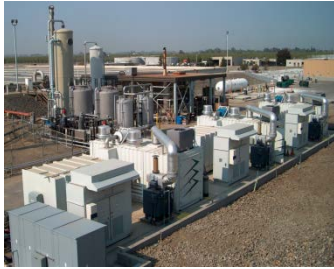
Tulare, CA, Municipal Wastewater Treatment Plant with fuel cells and ancillary equipment in foreground Photo from Frank Wolak, FuelCell Energy
