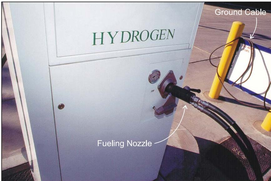
**Figure 7-8** Hydrogen Fueling Equipment at SunLine Transit Agency
