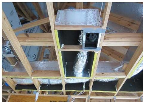
Insulated attic coffered were utilized in key locations to allow for the placement of ductwork in conditioned space without dropping the ceiling. This maintained the indoor aesthetic in rooms such as kitchens, living and dining areas, and wide open spaces.
