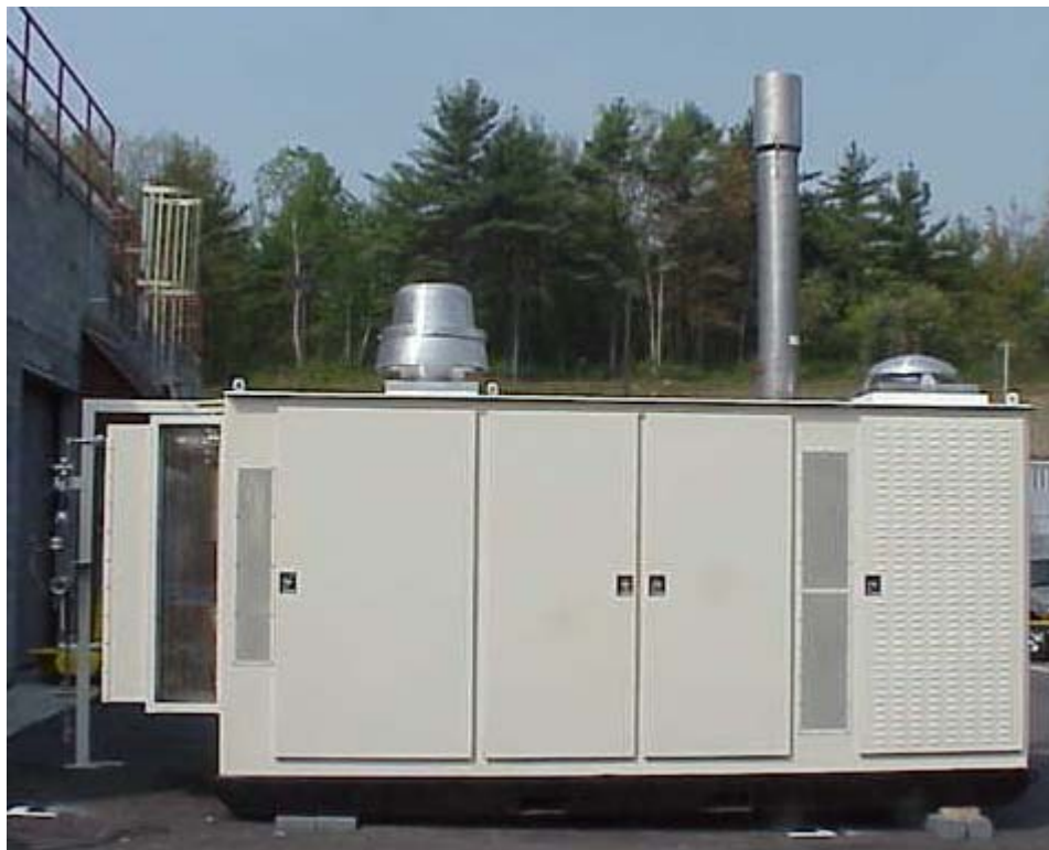
Figure 2: Plug Power Fuel Cell Power Plant
