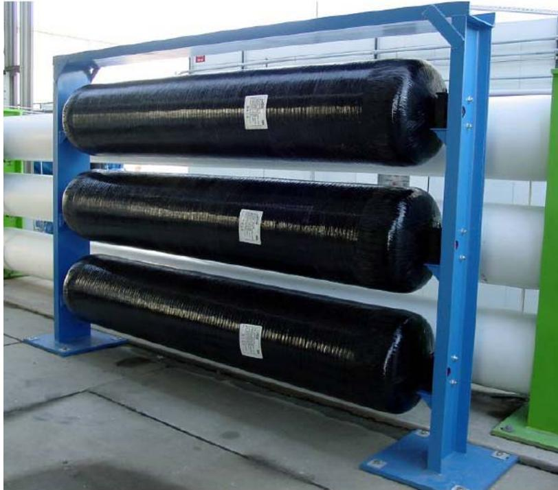
Figure 2-20 Cascade Storage Vessel Arrangement
