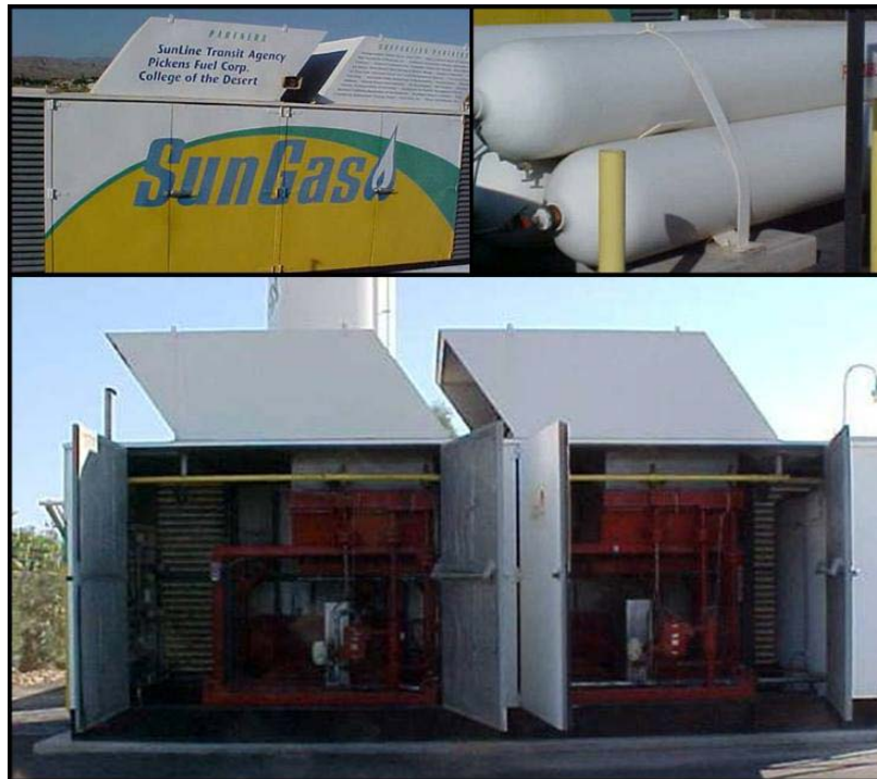
Figure C-3. CNG compressor station (Thousand Palms)
