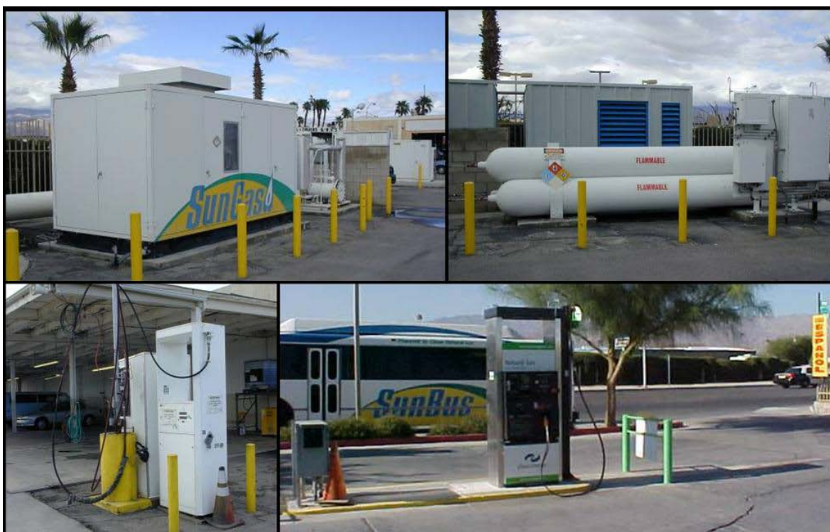
Figure C-4. CNG fueling equipment (Indio)
