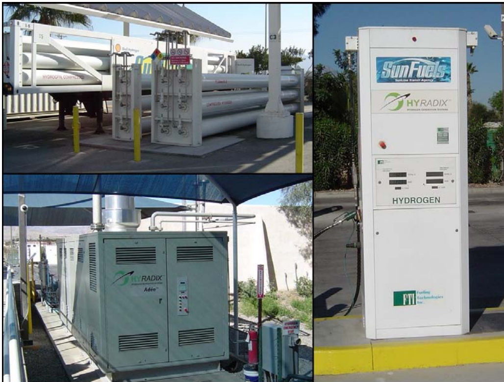
Figure C-6. SunLine's hydrogen storage (top left), HyRadix Adéo commercial reformer (bottom left), and hydrogen dispenser (right)
