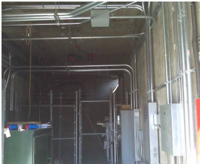
Figure 7. Energy monitoring node location for single-phase monitoring circuits.
