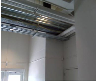
Figure 9. Conduit runs for the wireless mesh nodes.
