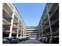
Figure 1. National Renewable Energy Laboratory's parking structure – open building design allows for daylight design. The design of the parking structure can affect the energy performance of the structure more than luminaire selection.
