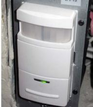
Aerosolized duct sealing (left) helped reduce duct leakage to outside by up to 62%. Lighting controls, like this occupancy sensor (above), helped to automate control and reduce energy consumption.
