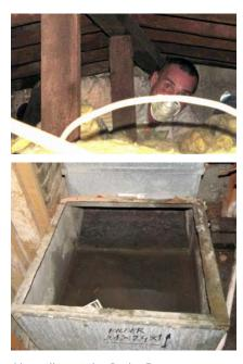
Air sealing at the Sasha Bruce group home in Washington, DC (top), required accessing some tight spaces. The existing plenum (bottom) had 4 in. of standing water from an improperly plumbed condensate line! Replacing and replumbing saved energy and improved indoor air quality.
