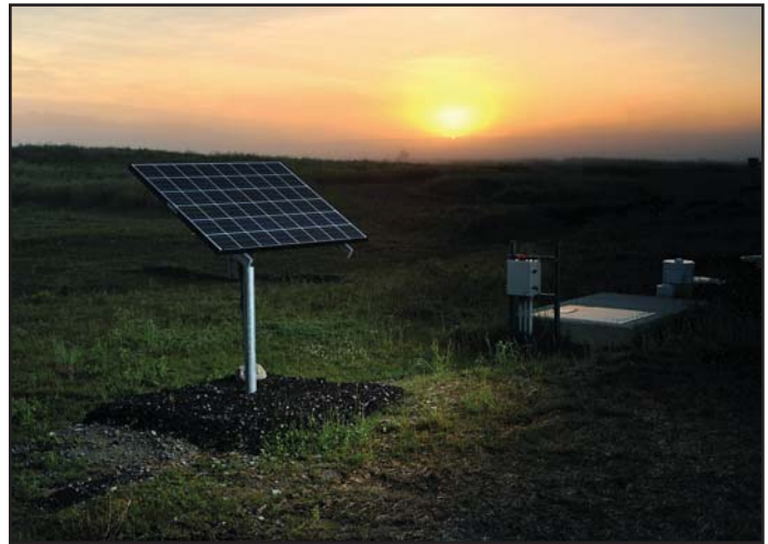
The solar panel that generates electricity to operate a pump for the Visitors Center's zero-discharge wastewater system.
