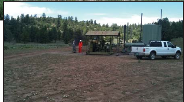
Gas wellhead apparatus including separator, condensate tank, condensate pump, and associated valving, at a natural gas well in the San Juan Basin near the Gasbuggy site in New Mexico.
