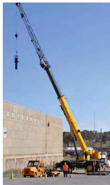
Sodium fluoride traps are removed through the roof of the K-25 Building at ETTP.
