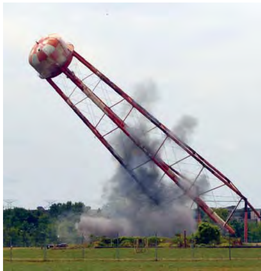
The water tower at ETPP comes down in a controlled demolition.
