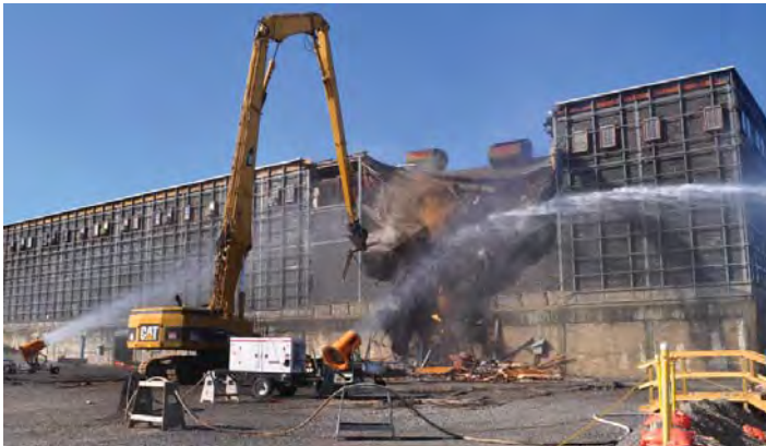
Demolition of the K-25 North Tower began in October 2012.
