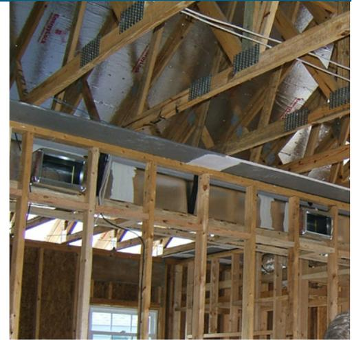
FSEC worked with Tommy Williams Homes of Florida to design a compact duct system with ducts located in dropped ceilings inside the home and supply registers coming directly off the trunk line wherever possible.
