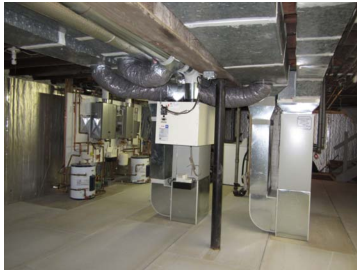
Rinnai RC80 HPI ODH Tankless Water Heater Rinnai 045 AHB Hydronic Air Handler (ECM fan)
