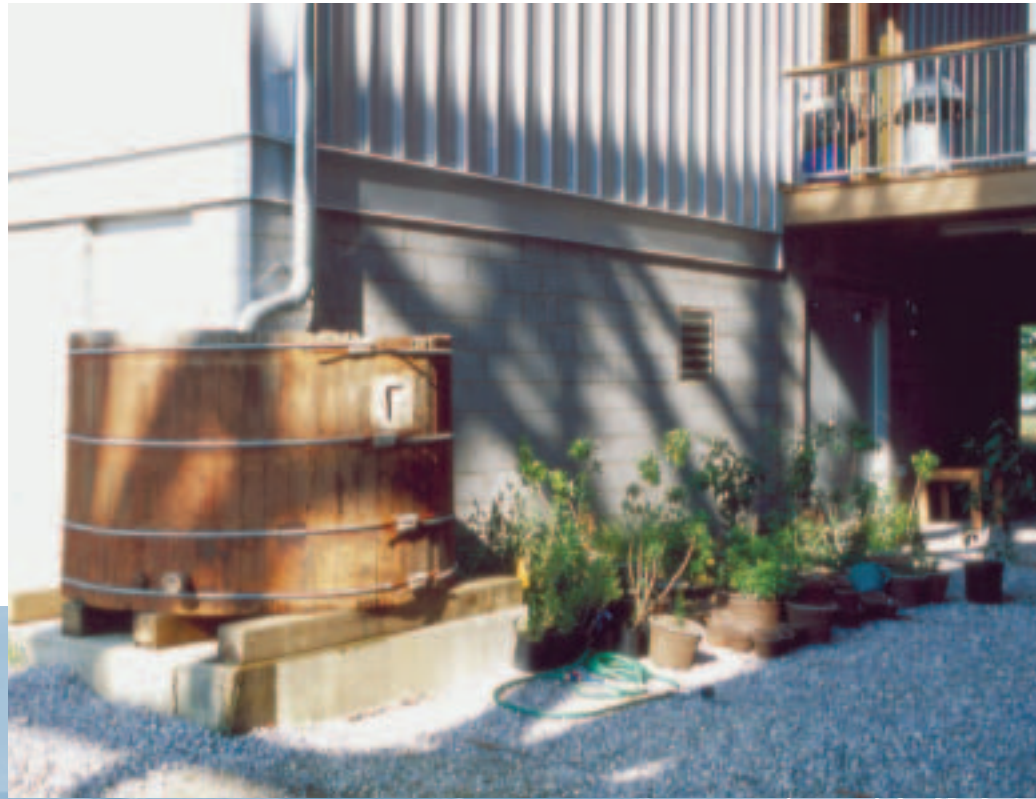
A small cistern stores rainwater for landscape irrigation at the Chesapeake Bay Foundation's Phillip Merrill Environmental Center in Annapolis, Maryland.
