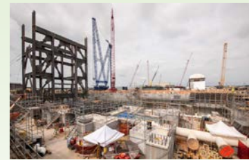
Vogtle Unit 4 Nuclear Island rebar placement and Unit 3 turbine support structure (Courtesy of Georgia Power/Southern Company)
