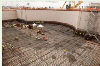
Vogtle Unit 4 Nuclear Island rebar placement and Unit 3 turbine support structure (Courtesy of Georgia Power/Southern Company)
