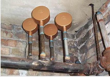
PARR upgraded the main line venting on steam mains in all of the test buildings. These vents allow steam to be distributed quickly and evenly throughout a building.
