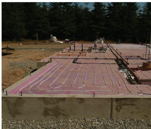
A ground-source heat pump heats water for the radiant floor heating loops in the first- and second-floor slabs. The heat pump also heats all of the home’s domestic hot water.
