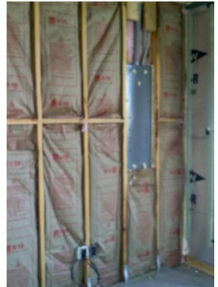
Inset stapling was used to fasten the insulation to the sides of framing, which created a thermal bypass. The builder restapled the kraft tabs to the stud faces to remedy this problem.
