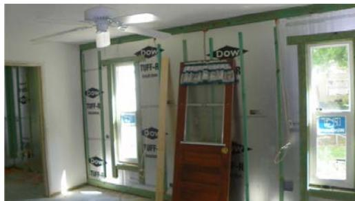
HFH removed old drywall and filled numerous holes in the concrete block walls before insulating them with continuous R-7.5 foil-faced rigid insulation. Borate-treated furring strips were attached over the insulation to provide an air gap behind the new drywall. (Photo Source: Calcs-Plus)
