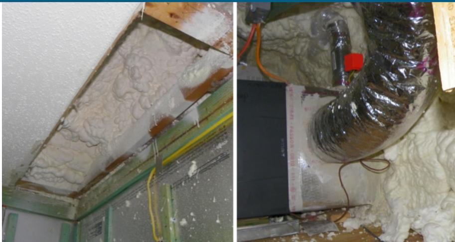
Ceiling drywall was removed along the perimeters of the home to access the attic. Open-cell spray foam was sprayed along the underside of the low-pitch roof to provide an R-21 air sealed, insulated attic space to house the new SEER 16.25 heat pump. (Photo Sources: Calcs-Plus)
