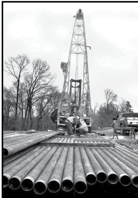
Workers prepare a well drilling site on the Oak Ridge Reservation. DOE and Bechtel Jacobs, Co., drilled a cluster of three wells at various depths to detect possible migration of contaminants from the Bethel Valley Burial Grounds.
