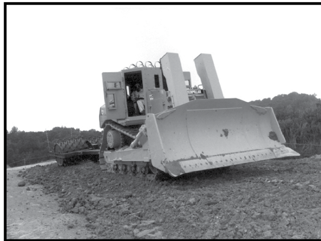
Bulldozers smoothed the ground over the Bear Creek Burial Grounds prior to the area being covered with a concrete cap.
