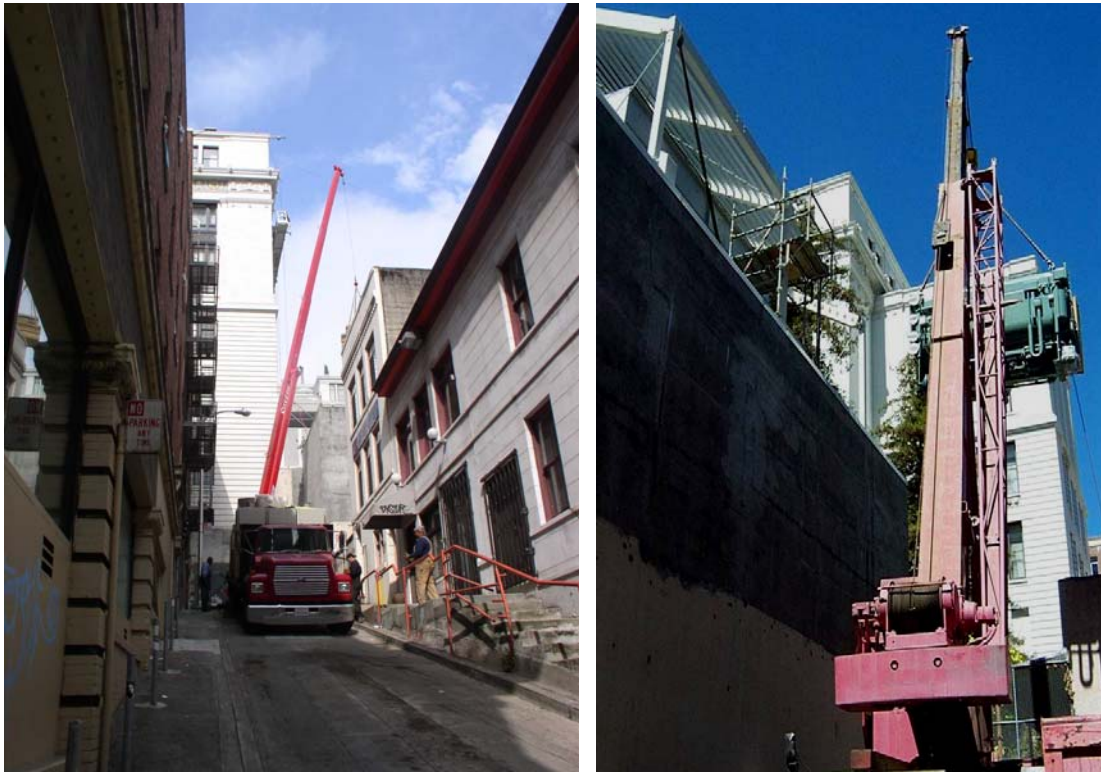
Figure 11 Hoisting the Chiller
