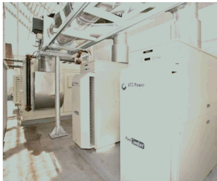
Figure 8 CHP System Layout on Ritz-Carlton Rooftop
