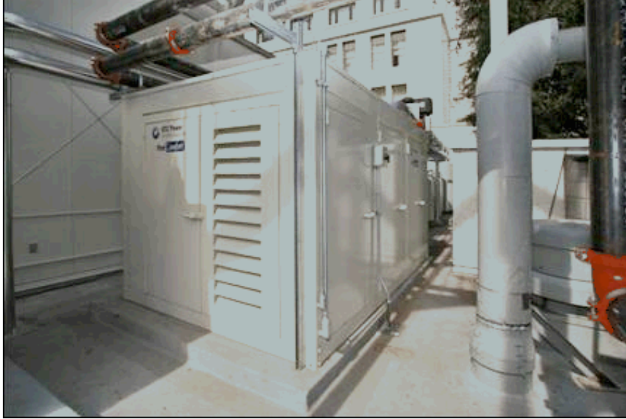
Figure 10 Installed Absorption Chiller with Enclosure
