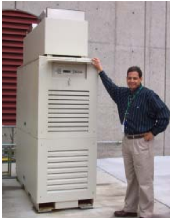
Capstone microturbine - 60 KW
