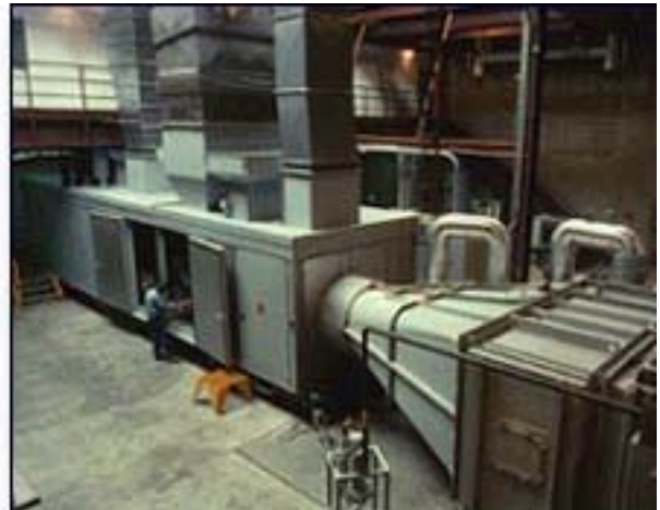
Figure 2-4. Rolls-Royce Allison 501-K Turbine Power Package
