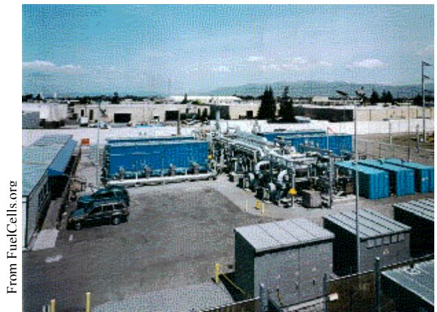
Figure 2-5. Fuel Cell Energy's 2 MW Molten Carbonate Fuel Cell power plant demonstration in Santa Clara, California
