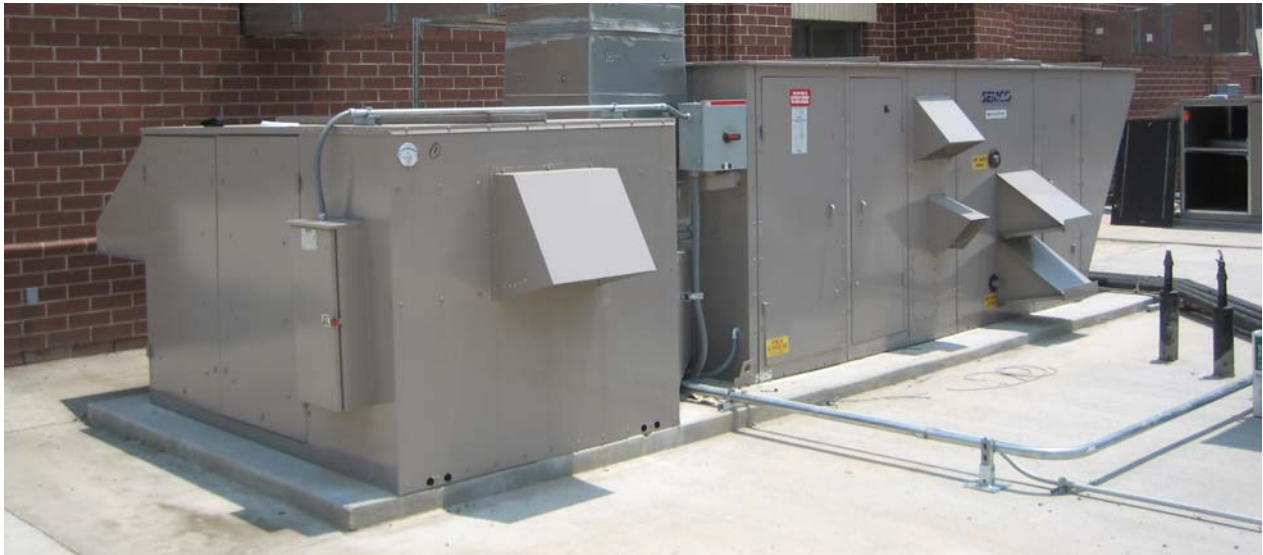
Figure 5. Photograph of the total energy recovery module matched with each IADR system.
