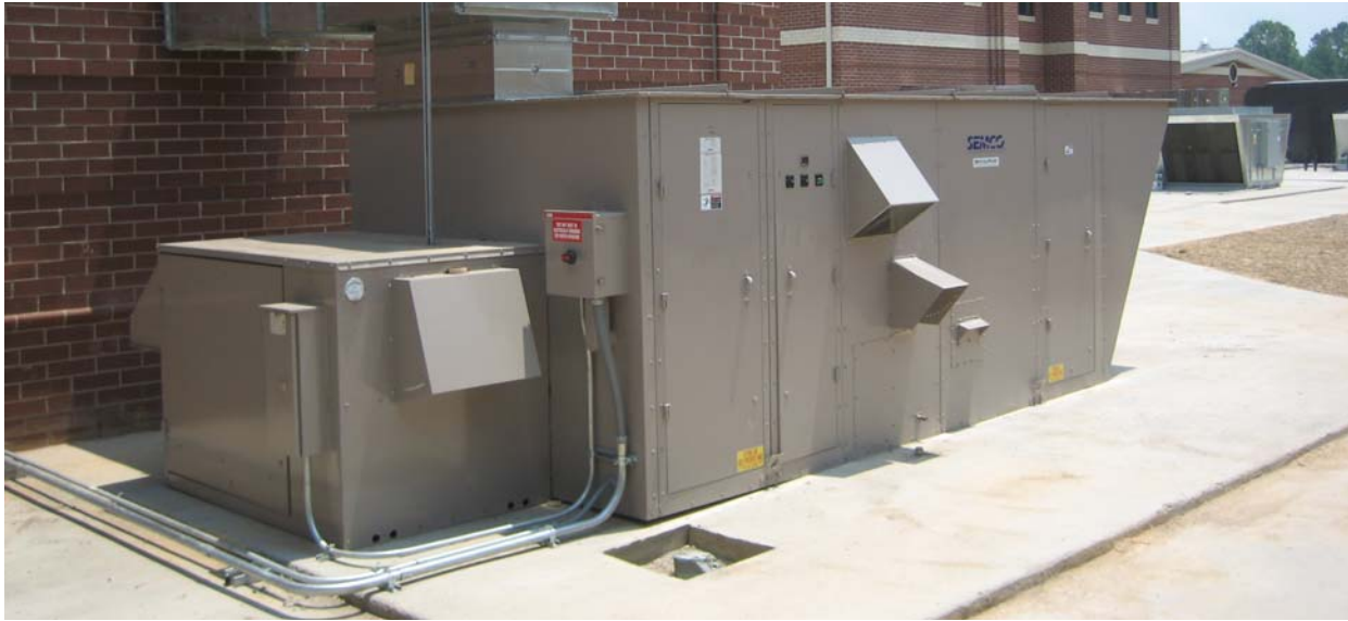
Figure 3. Photo of the IADR and total energy recovery module being installed at the research site
