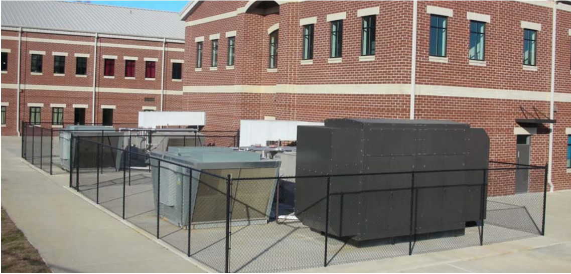
Figure 15. Photo of cogeneration package installed behind the Pepperell School
