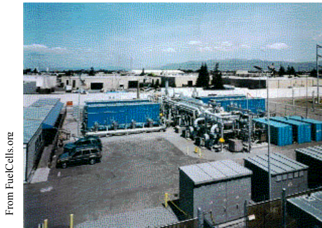
Figure 2-9. Fuel Cell Energy's 2MW Molten Carbonate Fuel Cell power plant demonstration in Santa Clara, California
