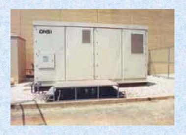
Fuel cells produce very few emissions (no combustion) and have high electric efficiencies (30-40%), but require more maintenance (2-4 cents/kWh)
