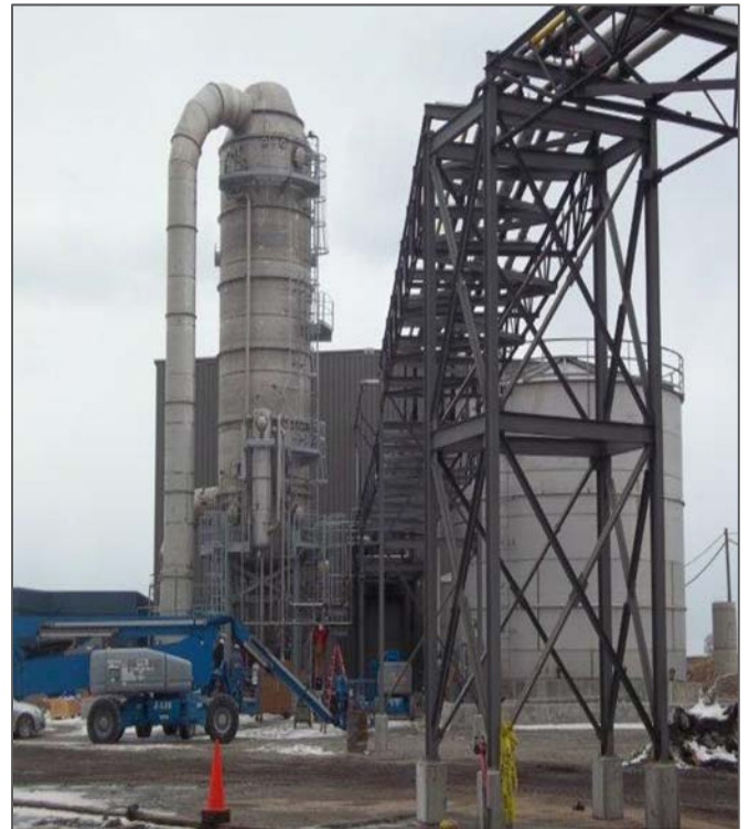
American Process, Inc. integrated biorefinery pilot plant in Alpena, Michigan
