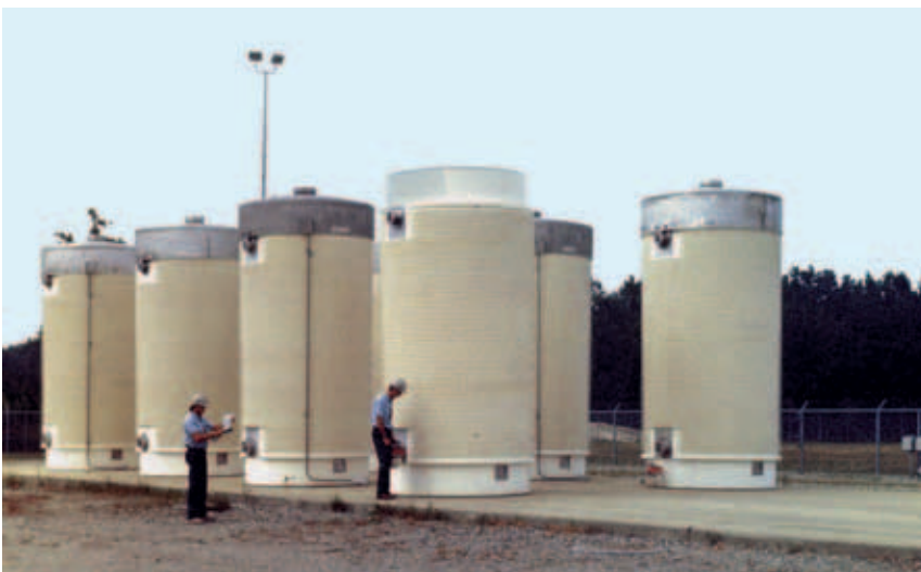
These dry storage casks hold spent nuclear fuel assemblies that have cooled for at least one year.
