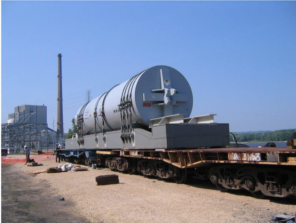
Figure 2-111. La Crosse Reactor Pressure Vessel on Rail Spur
