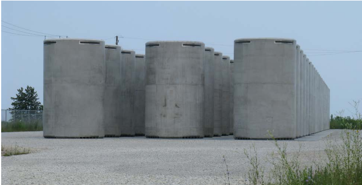
Figure 2-118. Vertical Concrete Storage Casks Staged at Zion
