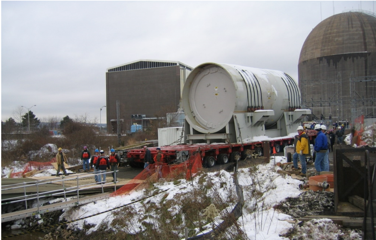
Figure 2-37. Connecticut Yankee Reactor Pressure Vessel Being Loaded onto Barge
