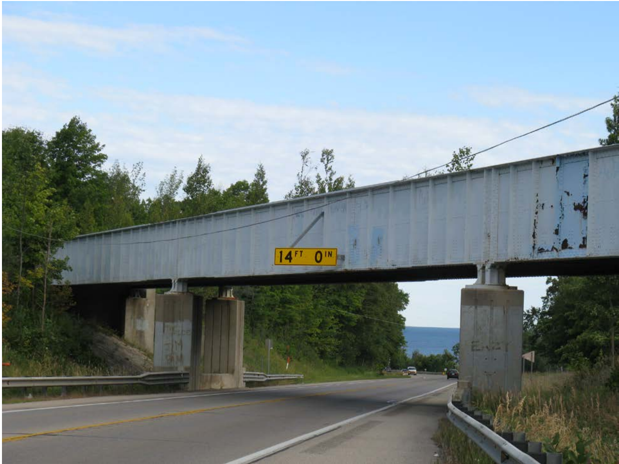
Figure 2-67. Low Overhead Clearance Abandoned Railroad Bridge
