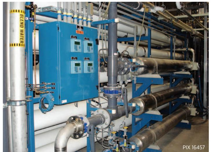
The HERO™ system consists of horizontal high-pressure pumps made of stainless steel that force spent water through a reverse osmosis membrane, which is inside the cylinder with the white housing.
