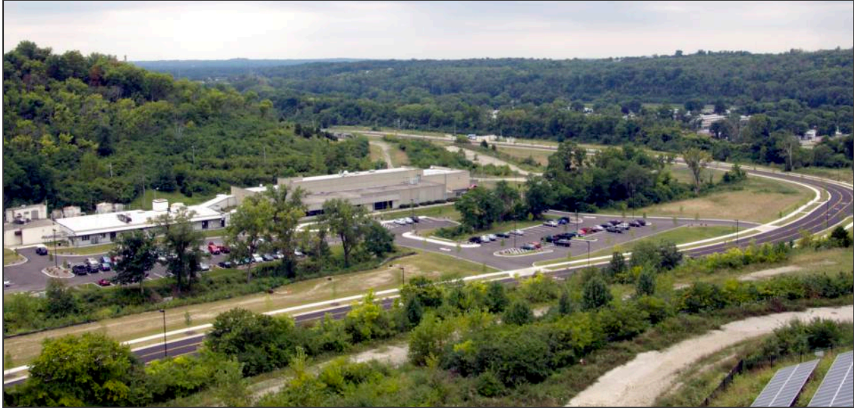
Improvements to the Mound Site property by the Mound Development Corporation included the construction of a roadway through the site which increases access to the various property plots, sidewalks, and parking lot upgrades.
