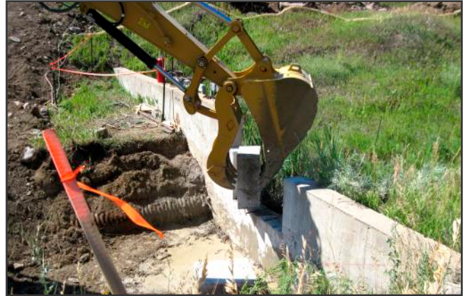
Construction contractors used heavy equipment to remove the sections of the diversion structure concrete that were sawn for the new notch.
