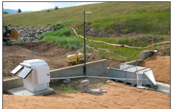
The new GS10 surface water monitoring location with automated sampling equipment installed. The coffer dam used to retain stream flows is visible to the left.
