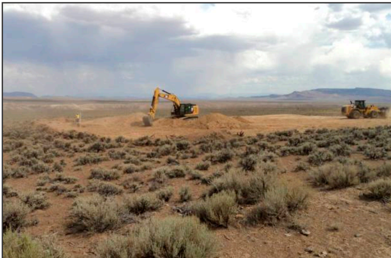
Initial grading and construction of the MV-6 well pad, Central Nevada Test Area, Nevada.
