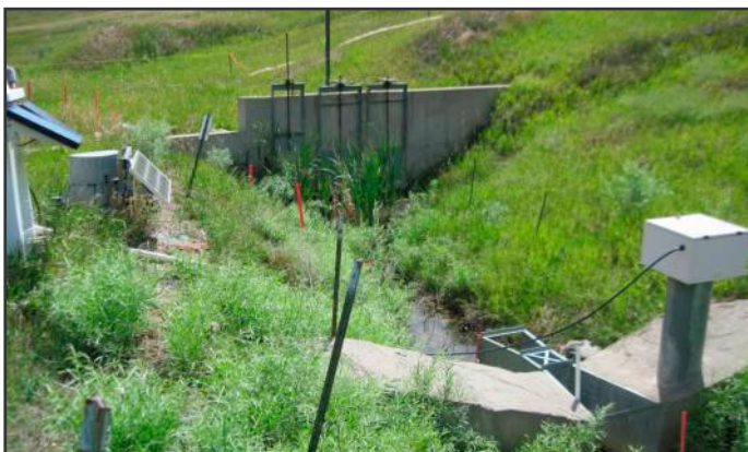
RFLMA POE sampling location GS10 and the downstream diversion structure prior to beginning the replacement project.
