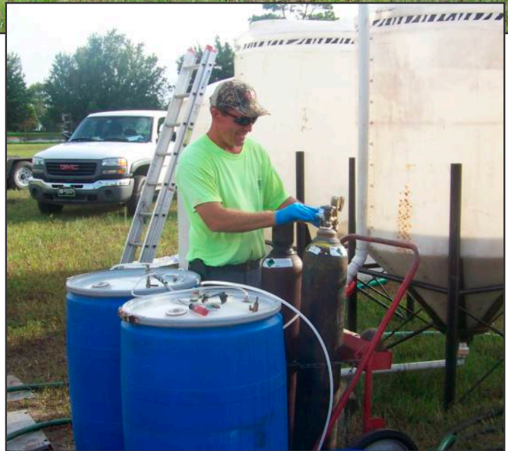
Top photo: A subcontractor uses a direct-push rig to inject the oil and microorganism mix.
