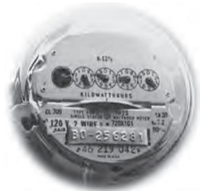
**Figure 8.1.1.** Typical utility socket-type meter
