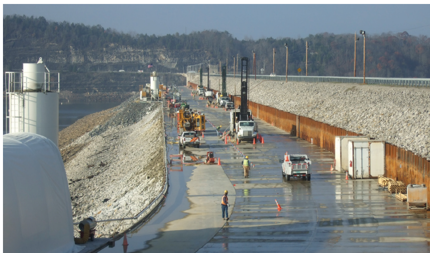
Nashville District contractors work on the Wolf Creek cutoff wall (Corps photo).
