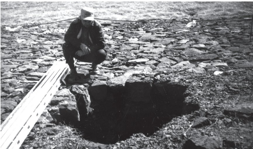
A sinkhole opened at Wolf Creek in 1968. This small hole represented big problems (Corps photo).
