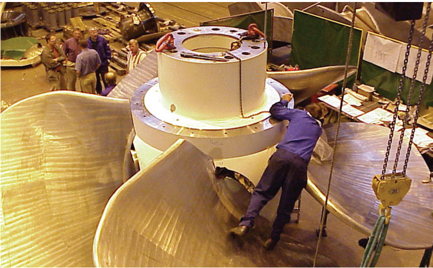
During the 1970s, the original variable pitch turbines at the Jim Woodruff project were periodically shut down due to severe vibration. In 2002, the Corps completed a major rehabilitation effort, greatly improving the plant's efficiency (Corps photo).
