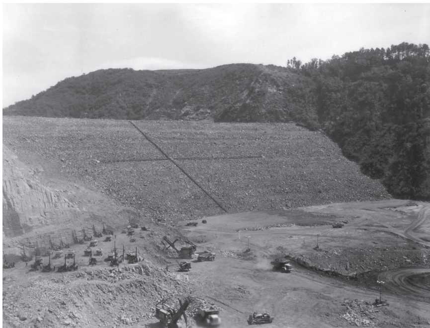
Construction on the Carters earth-filled dam required temporarily diverting stream flows through an adjacent mountain (Corps photo).
