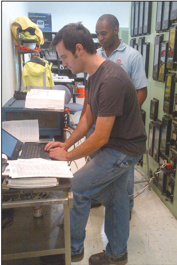
Electrical Engineers, Skylar Holloway, foreground, and Kellen Cole, verify and calibrate generator protective relay settings behind the Center Hill Powerplant control room switchboard.
