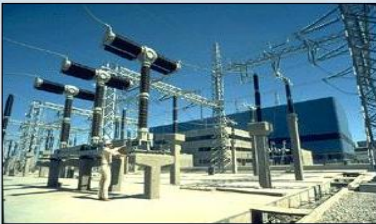
Figure 2. Step-up AC transmission substation
