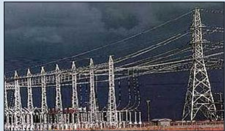
Figure 3. Step-up transmission substation to AC transmission lines
