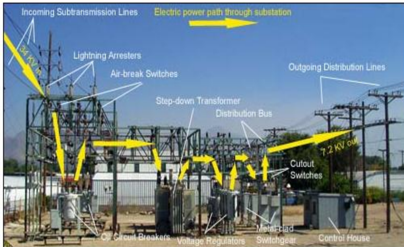
Figure 1. Typical substation
