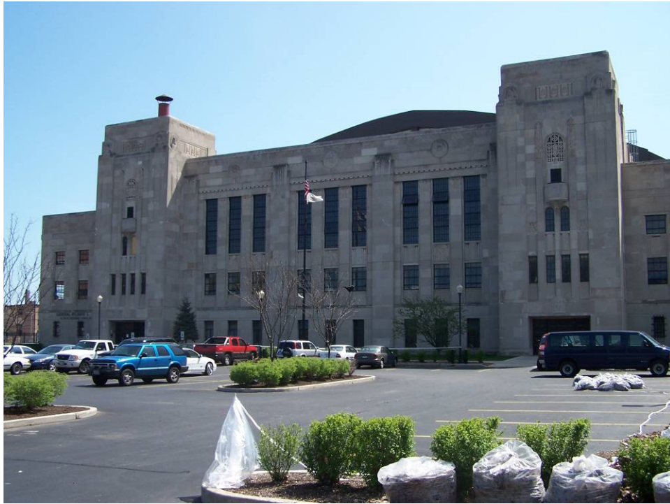
Chicago North, IL, site, April 2006
