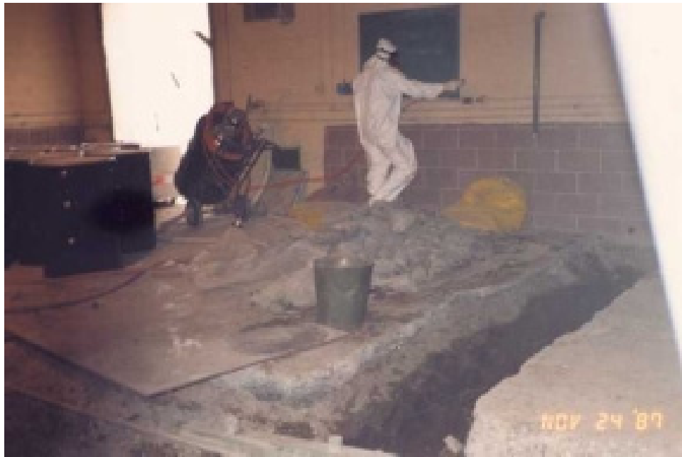
Scrubbing and sanding at Building 31, Albany, OR, site (DOE Digital Archive)
