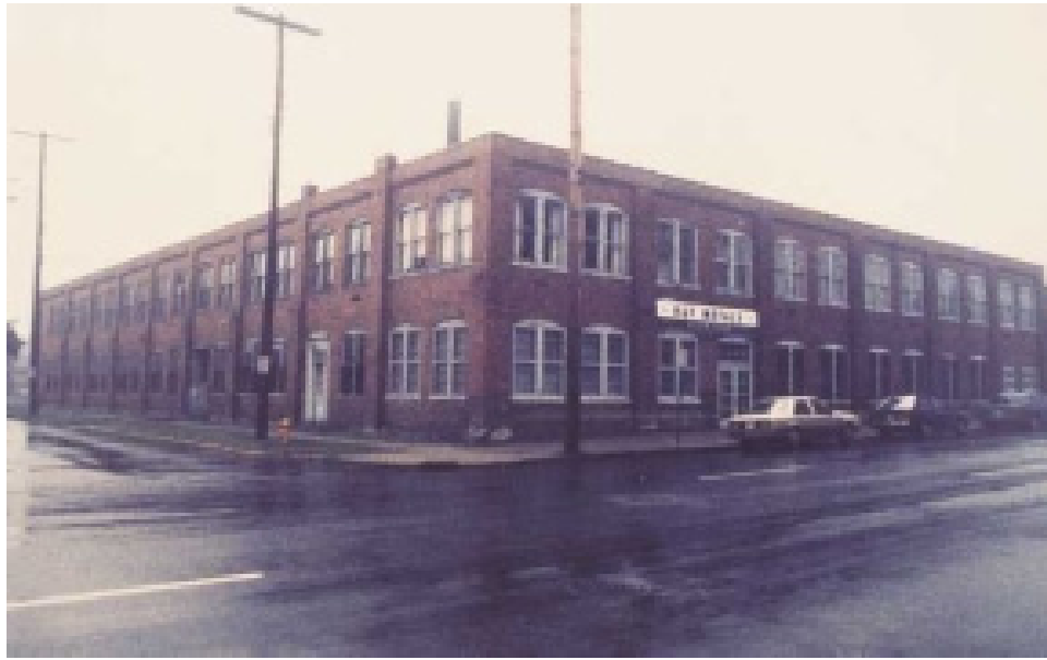
Columbus East site (B&T Metals), January 1995; most contamination was in the right (northwest) corner of the building (DOE Digital Archive)
