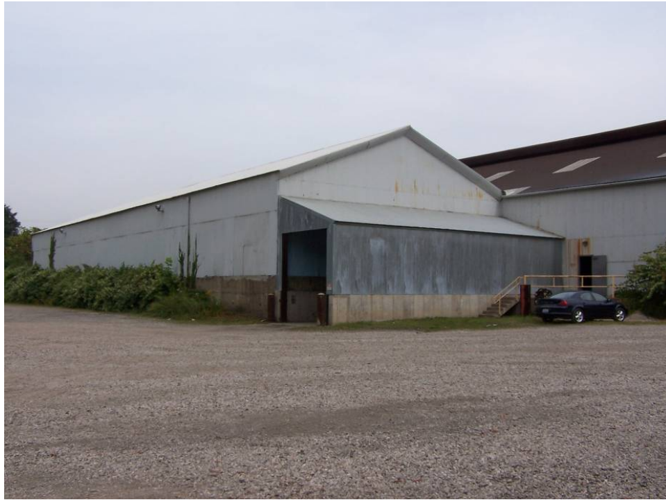
Front of remediated building in which AEC work occurred, Aliquippa, PA, site, September 2005
