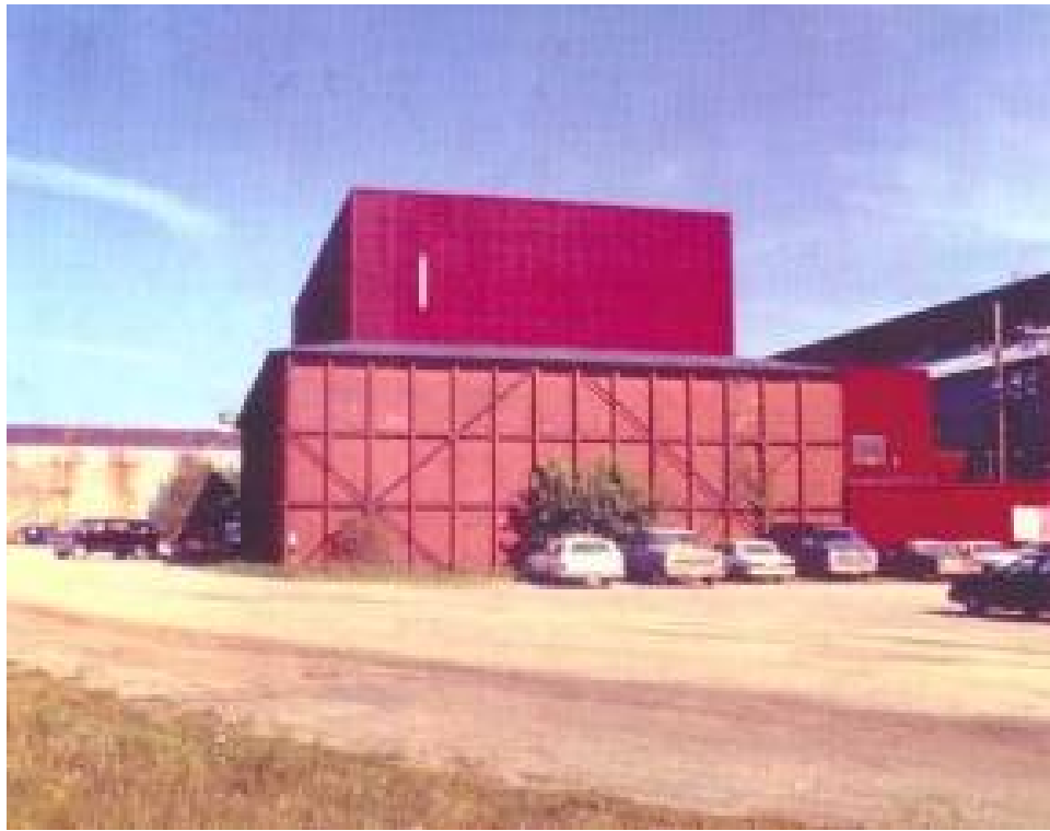
Betatron building at the Granite City, IL, site before remediation was conducted, 1991 (DOE Digital Archive)
