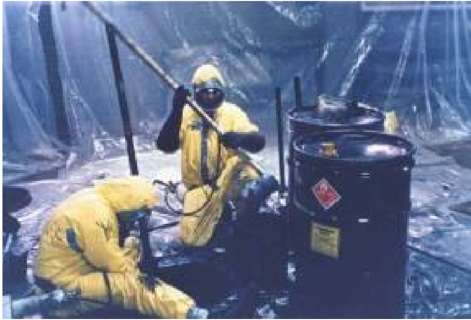
Removing sludge and placing in drums at National Guard Armory, Chicago North, IL, site, September 1987 (DOE Digital Archive)
