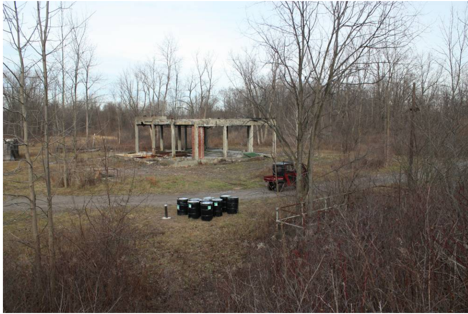
Abandoned wastewater treatment plant on Niagara Falls Vicinity Properties site, VP-X, December 2009 (USACE uses the drums to store purge water while awaiting analytical results)
