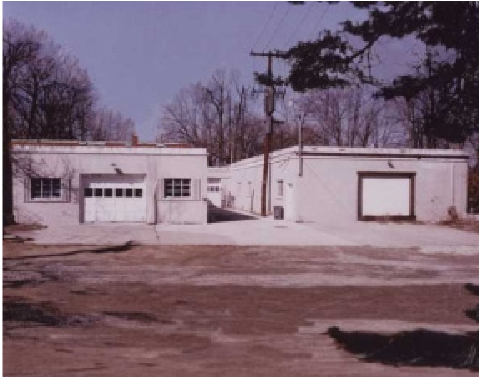
The Alba Craft Laboratory building before remediation (DOE Digital Archive)
