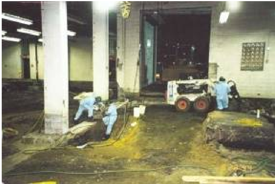
Remediation of C.H. Schnorr building interior, Springdale, PA, site, September 1994 (DOE Digital Archive)
