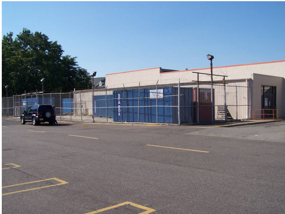
Jersey City, NJ, site in October 2007 showing the location where underground oil tank was to be removed; (records indicated this area was unaffected by FUSRAP contamination)
