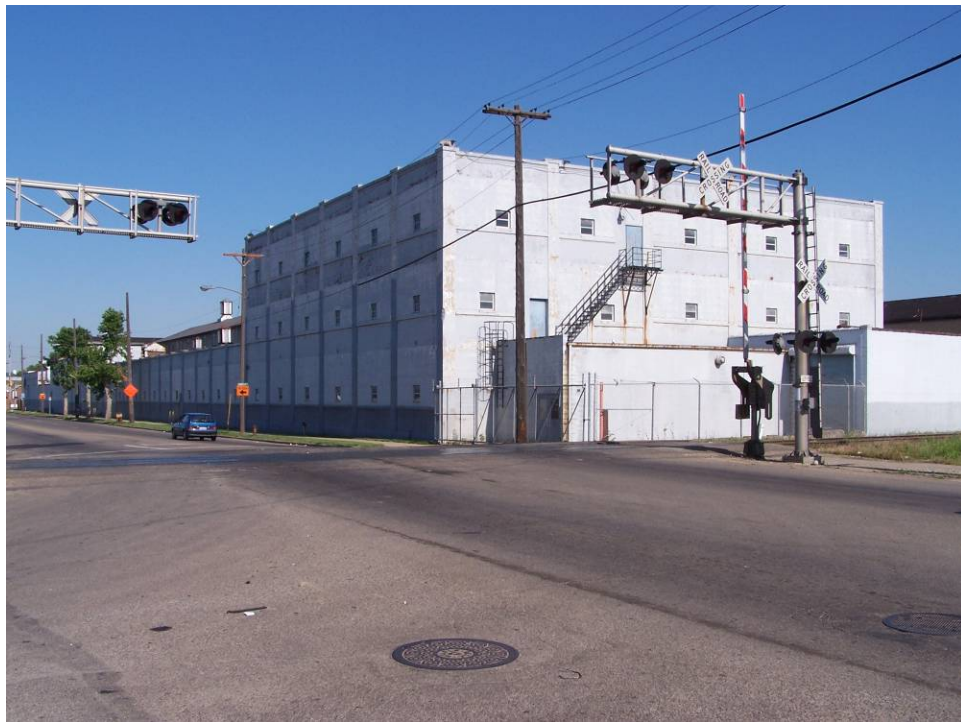
The Hamilton, OH, site in June 2006, showing third floor where FUSRAP remediation occurred
