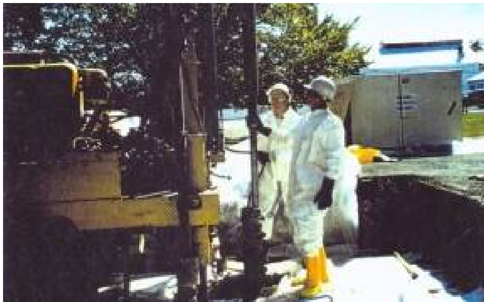
Radiological survey support work at the Albany, OR, site, December 31, 1991 (DOE Digital Archive)
