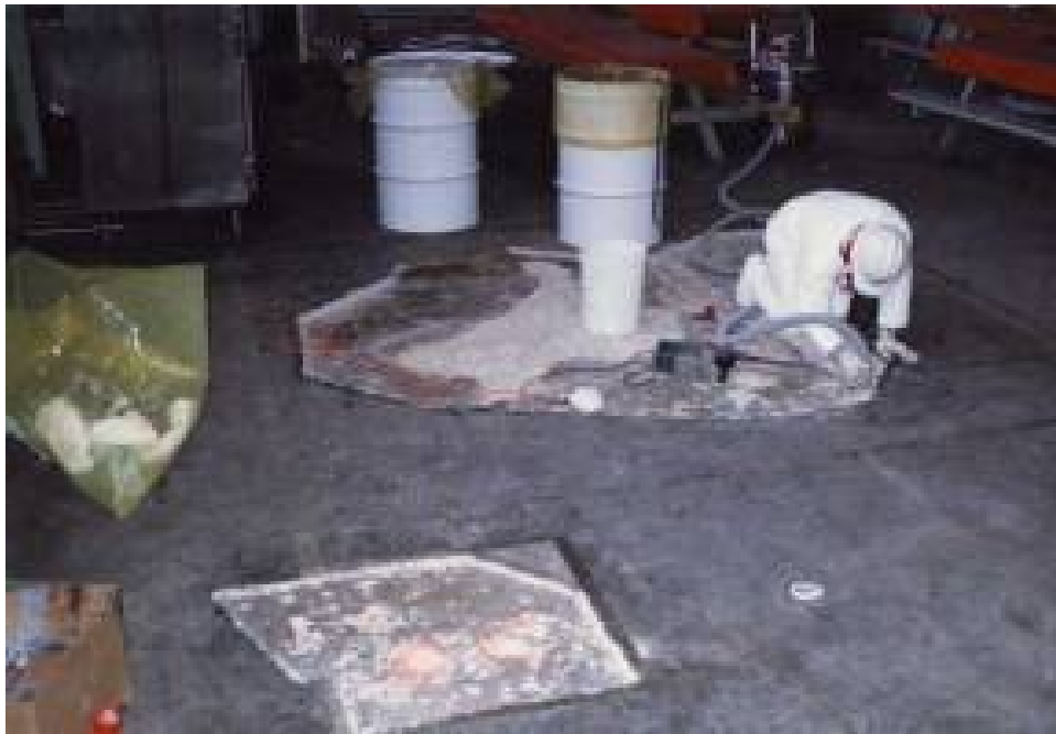
Scabbling concrete at National Guard Armory, Chicago North, IL, site, September 1987 (DOE Digital Archive)
