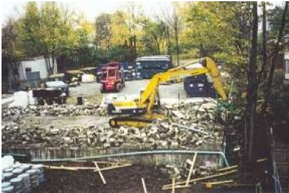
Demolition of the Alba Craft Laboratory building, October 1994 (DOE Digital Archive)
