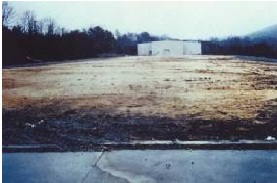
Oak Ridge Warehouses site after remediation, December 1992 (DOE Digital Archive)
