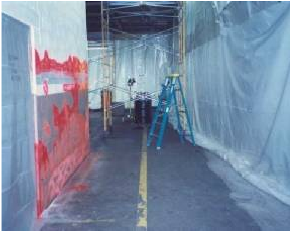
Interior remediation at the Fairfield, OH, site, December 1994 (DOE Digital Archive)
