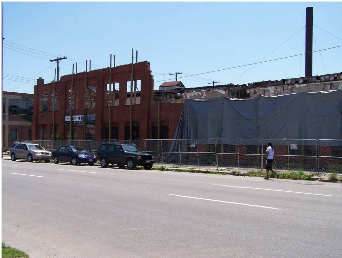
Former B&T Metals Building, June 2006
