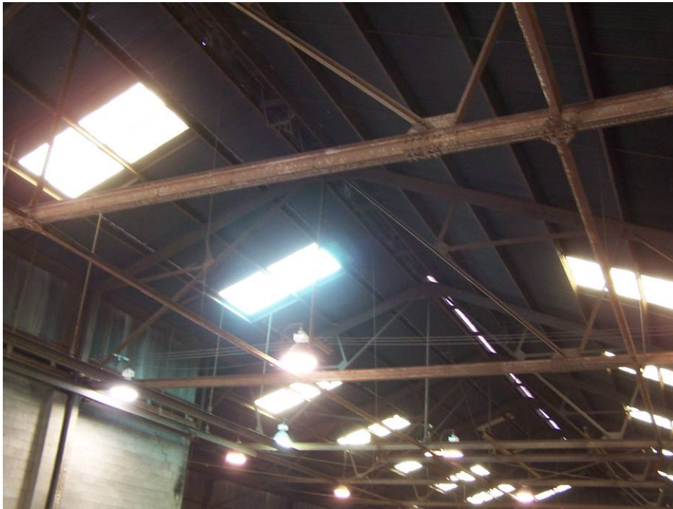
Roof system where supplemental limits were applied, Aliquippa, PA, site, September 2005
