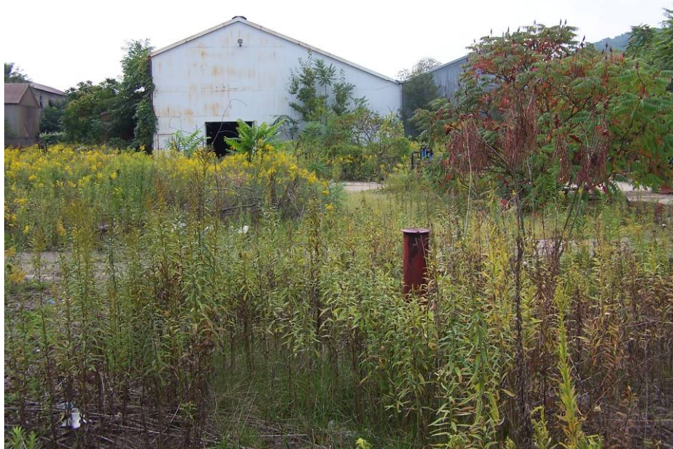
Rear of remediated building, compressor building foundation in front of building left of the open door; well in foreground was later abandoned, Aliquippa, PA, site, September 2005
