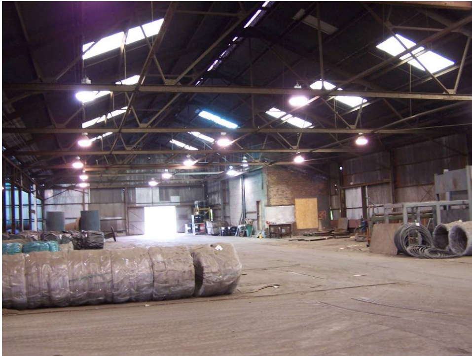
Building interior, Aliquippa, PA, site, September 2005
