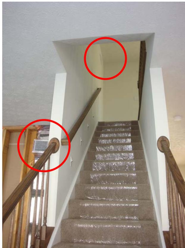
Figure 6. First-floor (left) and second-floor (top) supply register locations
