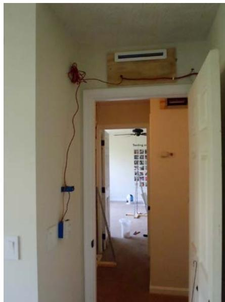
**Figure 5. Over-door powered transfer fans to bedroom 2**
