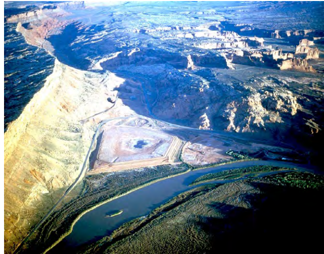
DOE responded to public and other agency concerns about the potential for the Moab tailings pile (center) to contaminate the Colorado River.
