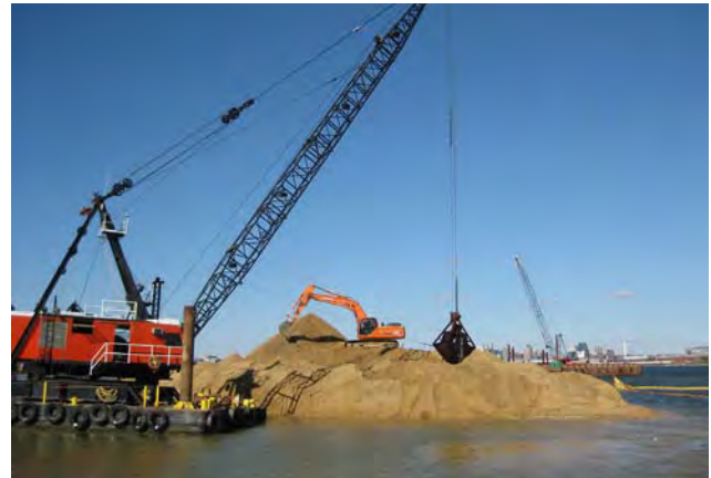
In 2007, the Maryland Port Administration began construction of the containment dikes for the Masonville Dredged Material Containment Facility. (photo: Kaitlin McCormick)
