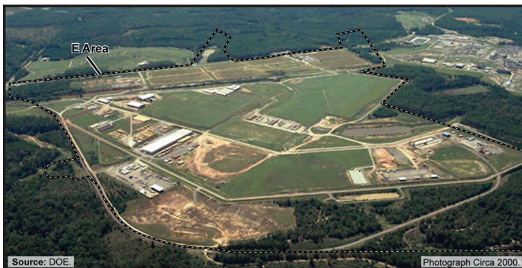
Figure 2-21. E Area at the Savannah River Site
