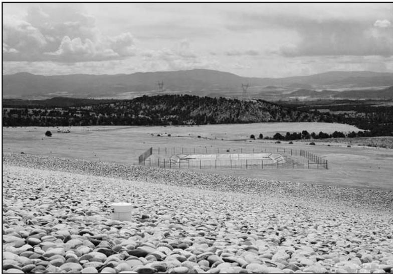
*Transient drainage water is pumped from the Rifle, Colorado, Disposal Cell to an evaporation pond.*
