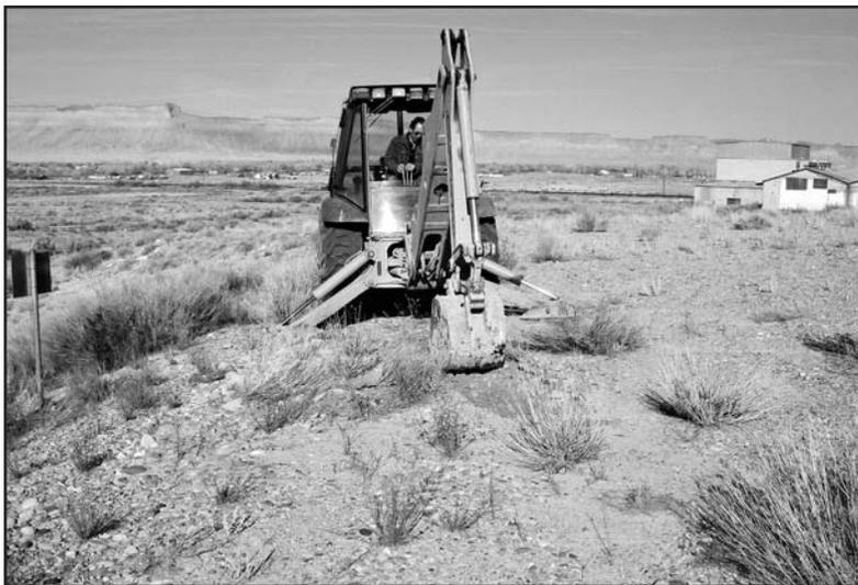
*Erosion repair was necessary to protect a perimeter sign at the Green River, Utah, Disposal Site.*
