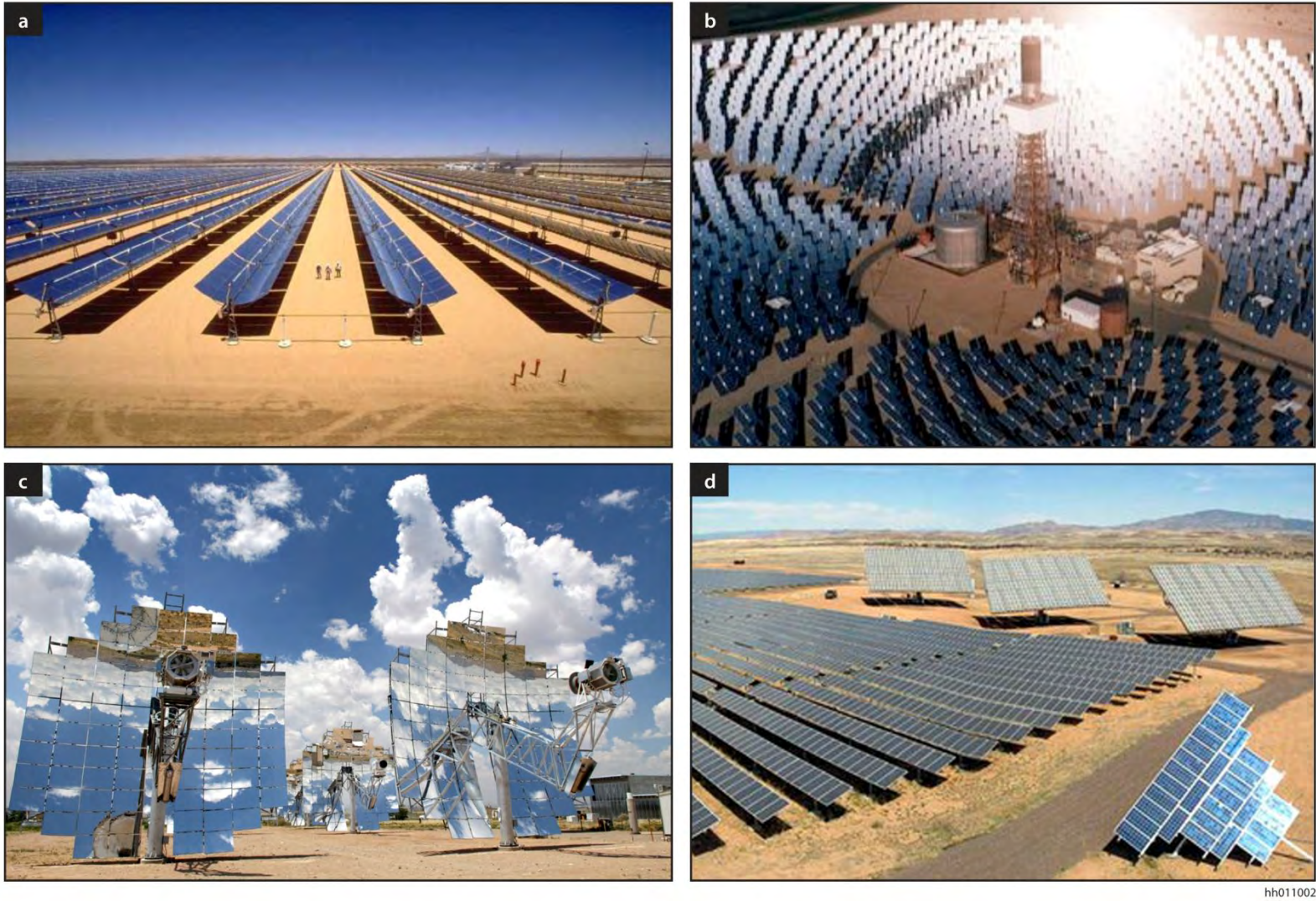
FIGURE 1.2-1 Typical Solar Fields for Various Technology Types: (a) Solar Parabolic Trough (Source: Hosoya et al. 2008), (b) Solar Power Tower (Credit: Sandia National Laboratories. Source: NREL 2010a), (c) Dish Engine (Credit: R. Montoya. Source: Sandia National Laboratories 2008), and (d) PV (Credit: Arizona Public Service. Source: NREL 2010b)
