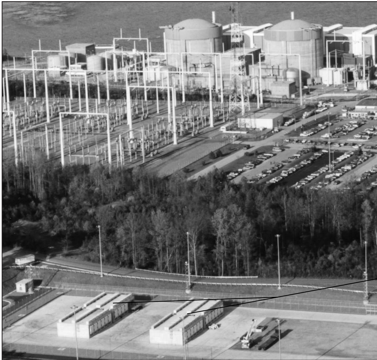
Figure 7-2. Typical independent spent fuel storage installation.
