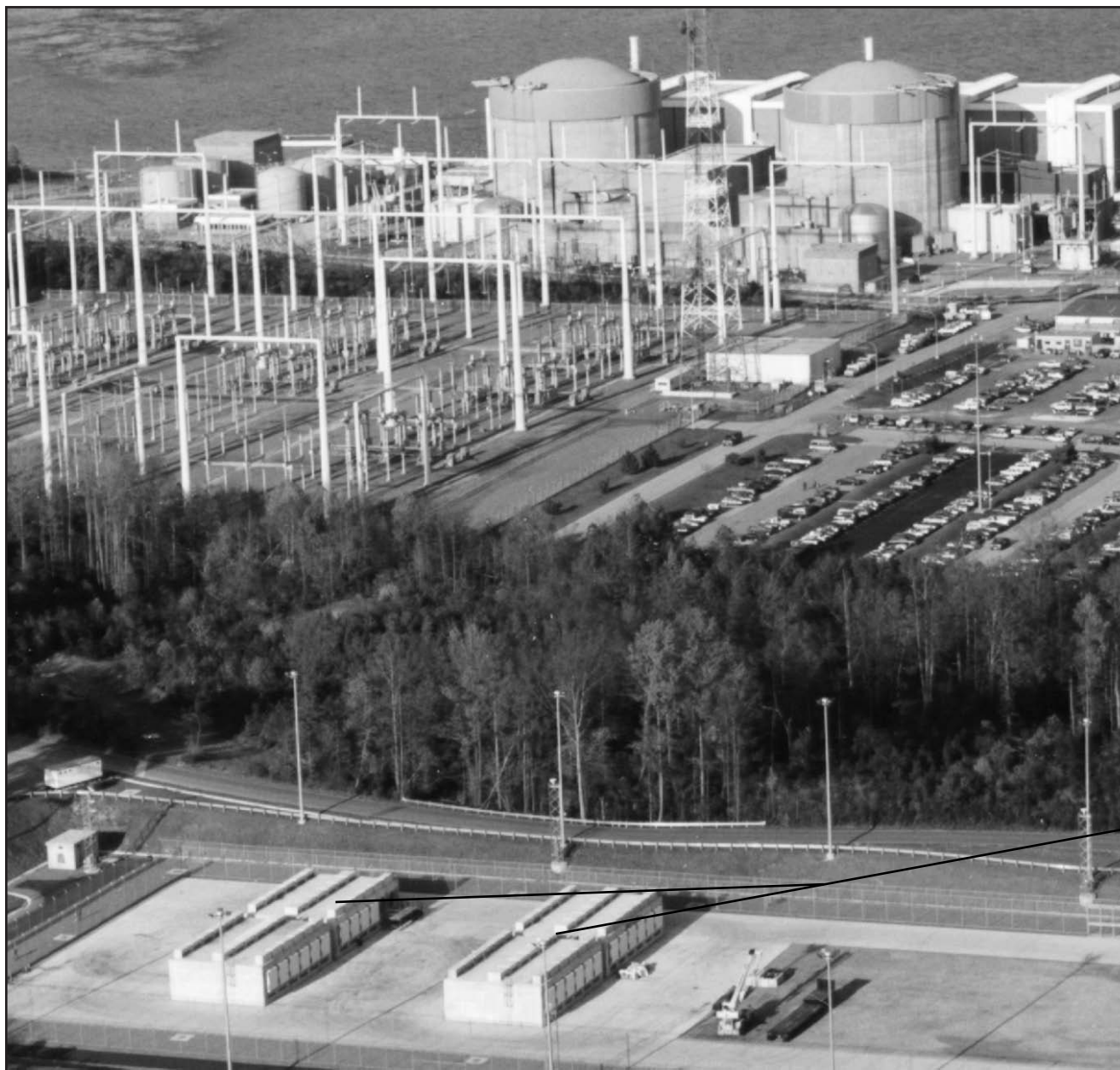
Figure 2-32. Typical independent spent fuel storage installation.
