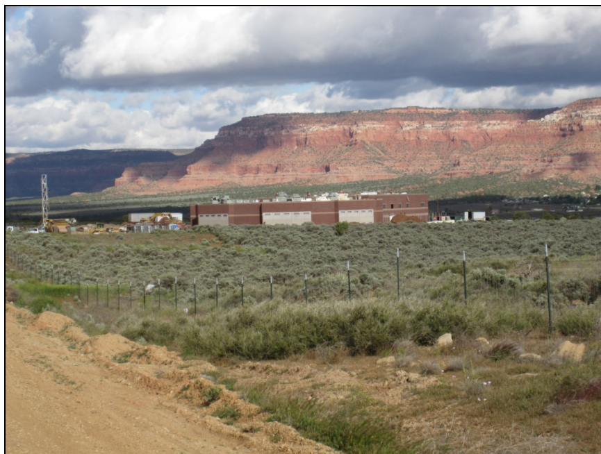
Figure 3-1. Kane County Public Safety Facility Construction, looking Northwest from Kaneplex Road
