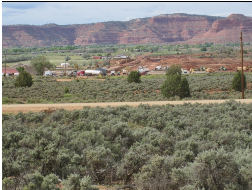
Figure 3-6. Telephoto View of Jackson Flat Water Supply Storage Project Construction from Proposed Pilot Plant Site
