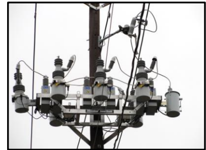
Switched Capacitor Banks
