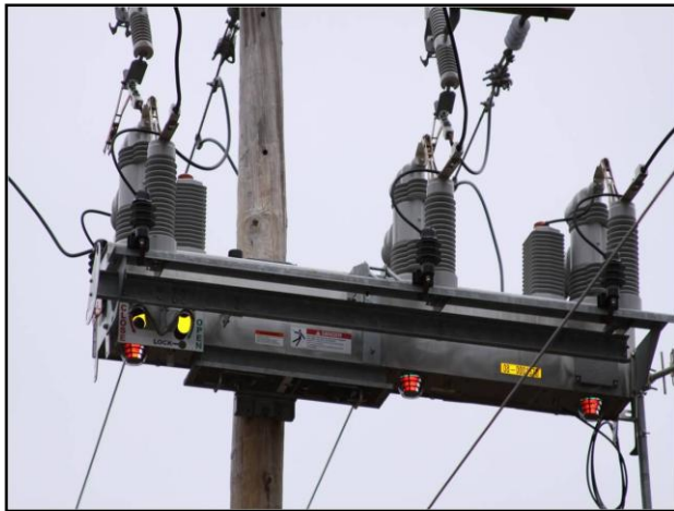
Smart switches installed in EPB service territory
